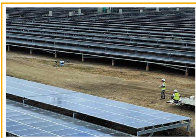
▲ Photo: Using of drone for module cleaning process for difficult to access sites
